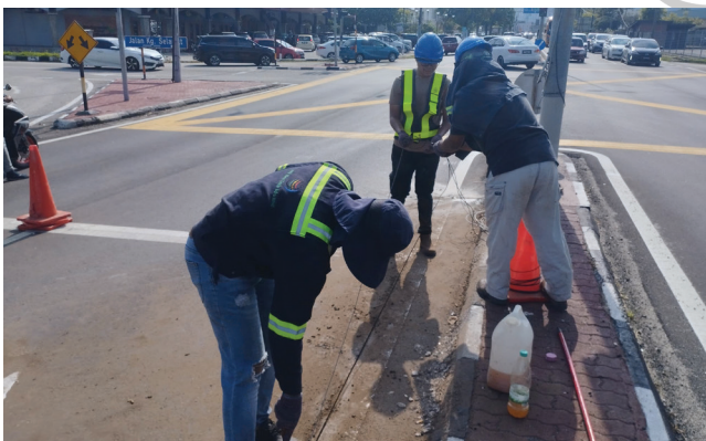
Loop sensor Installation Process
