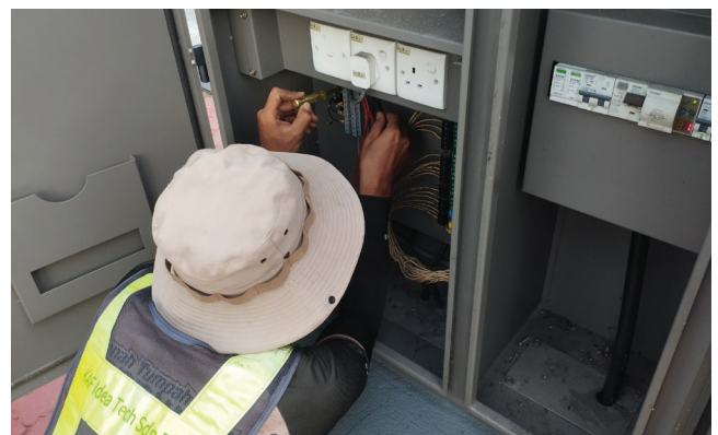
Wiring and termination for loop sensor
