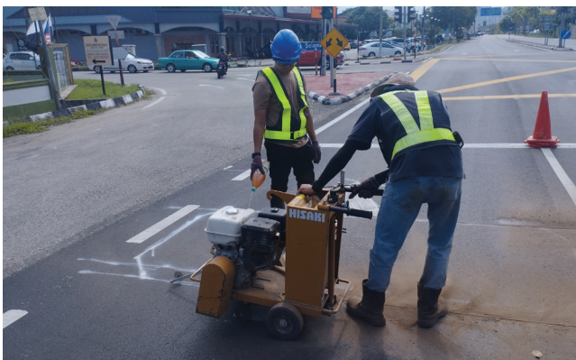
Loop sensor Installation Process
