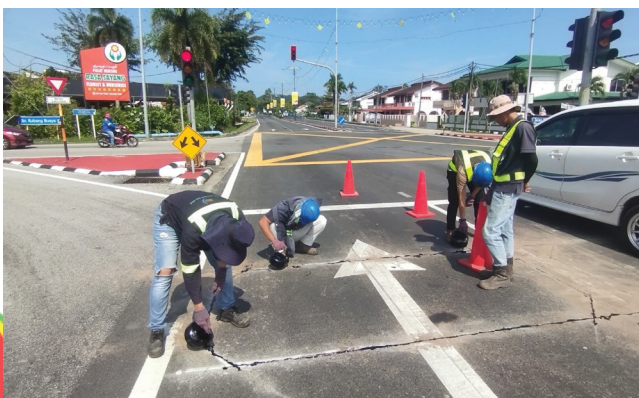
Loop sensor Installation Process
