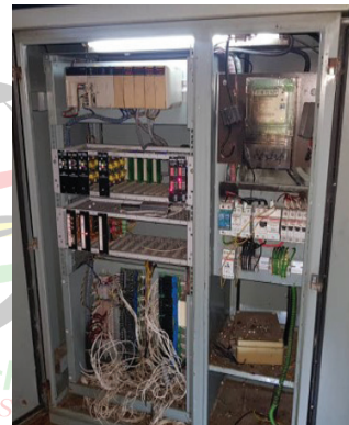
Upgrade old traffic light system to KAF iTAC Controller
