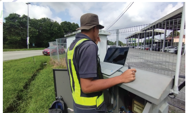
Setting loop sensor
